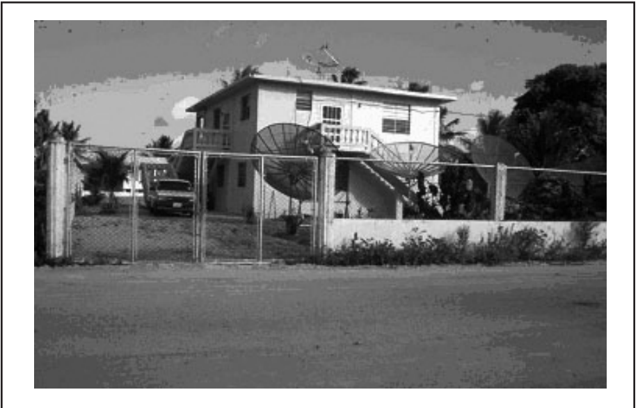
Figure 10. Hopkins television office.
