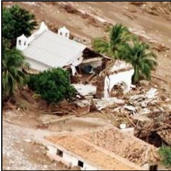
Fig. 5-188. The destroyed church 1998.
